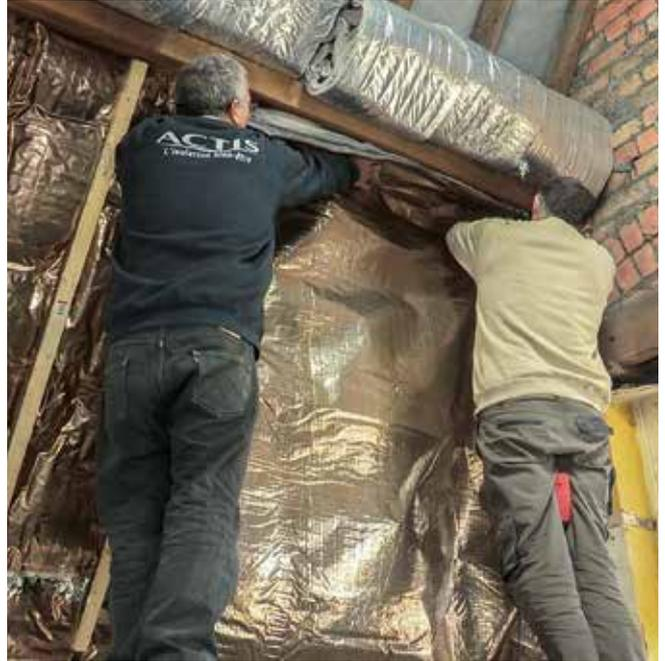
**3** Staple to timbers every 50mm as taut as possible, using 20mm galvanised staples. Cut **HCONTROL HYBRID** oversized at eaves and pitch, allowing it to be adequately sealed by a batten.
