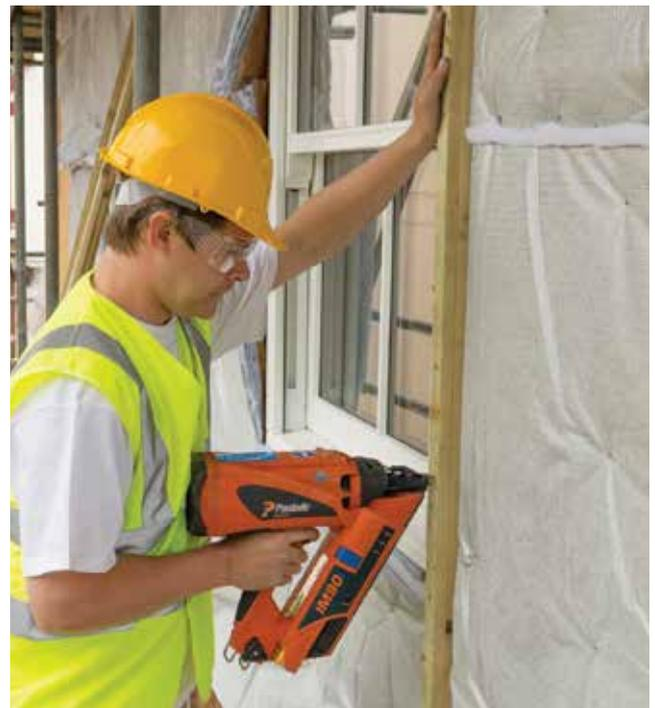
The installation requires careful detailing around doors and windows to achieve a satisfactory surface for finishing. In addition, make sure to minimise the risk of thermal bridging at reveals and where separating walls are attached to the external wall.
